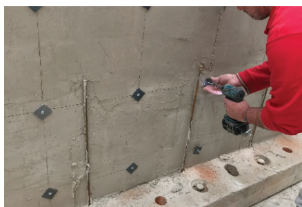
Pic 2: Steel rebar to connect plaster to foundation and connector application sample
